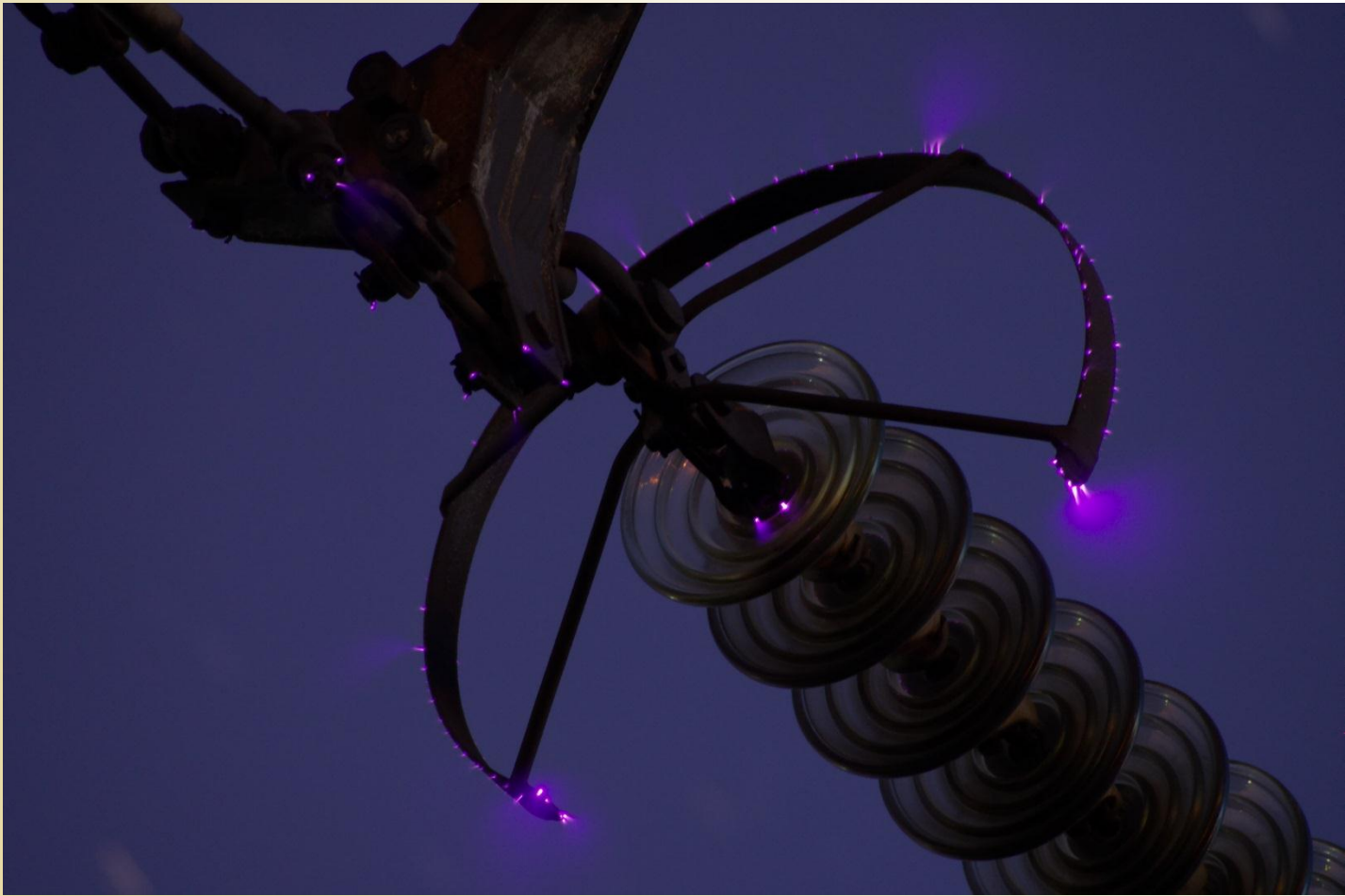
Corona Emission from Energized Parts of Transmission Line Suspension Insulator
