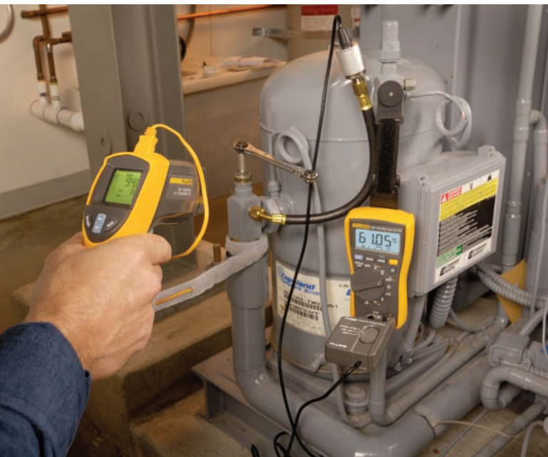
Measuring temperature and suction pressure to determine superheat.
