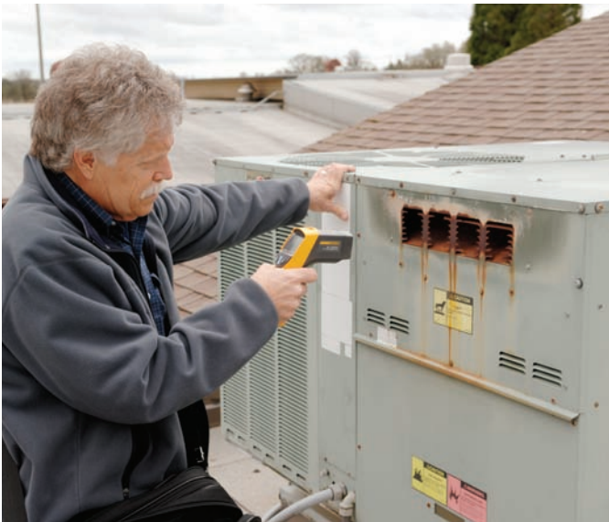
Testing roof-top refrigeration system with a Fluke 561 Infrared Thermometer.
